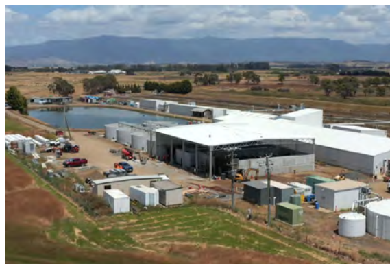
CRESSY III DURING THE CONSTRUCTION PHASE.
