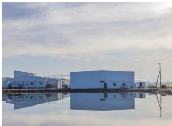
CRESSY III CONSTRUCTION COMPLETED AND ALL SHIP SHAPE.
